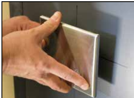
Tip - Use a piece of double-sided tape to hold the Exterior Trim Plate into place
