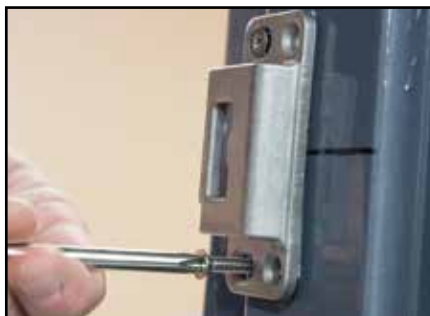
18e - Secure strike to the frame with (2) screws in the slotted holes
