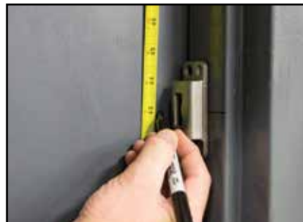
2a - Make multiple marks across the door at 43" from the finished floor
