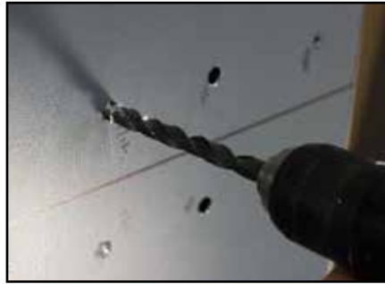
8a - Base Plate side of the door drill all (4) Exterior Trim B attaching holes
