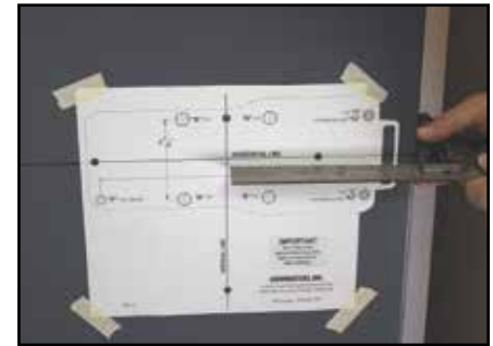
4a - Align combination square with Base Plate Template's vertical line.
