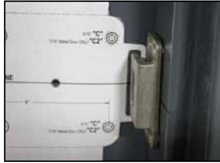
3a - Align Base Plate Template around Strike
