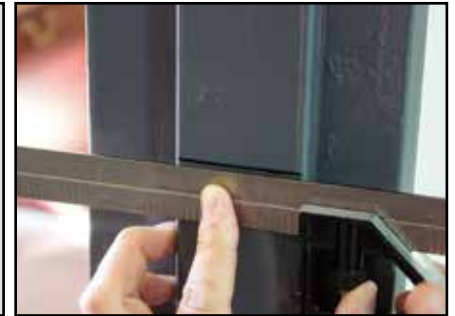
1b - Make a straight line across door frame
