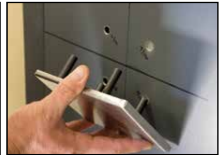
11a - Insert the Exterior Trim Plate’s stand-offs into the (4) B holes on the front side of the door.
