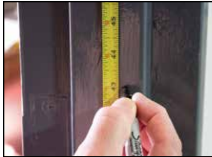
1a - Position strike at 43" above finished floor
