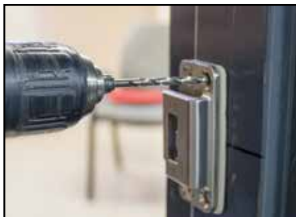
18h - Drill Pilot Holes in the remaining (3) strike holes and tap.
