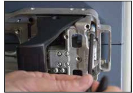
14b - Align Base Plate with drilled holes and secure to the door with 1/4"x20-1-1/4" socket head screws into (2) front C2 holes.
