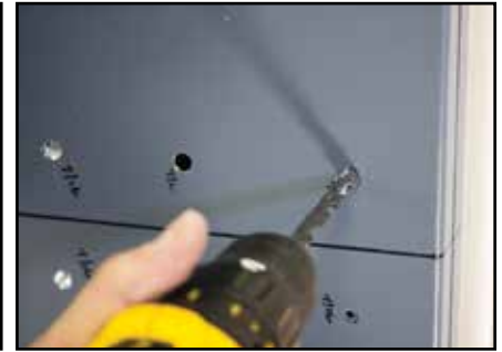
8b - Base Plate side of the door drill both Base Plate attaching holes (C2 for metal)
