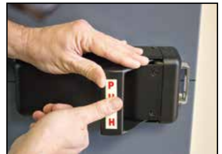
17b - Place the correct Pull or Push label on the Base Plate Handle
