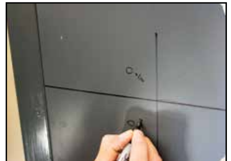
6d - Label all hole diameters from the template to the corresponding holes on the door
