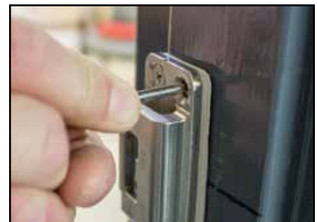
18h - Once in position Center Punch remaining (3) holes.
