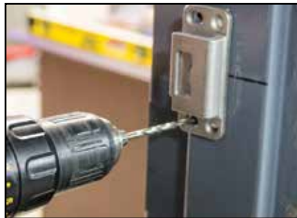
18c - Drill Pilot holes with #25 drill bit
