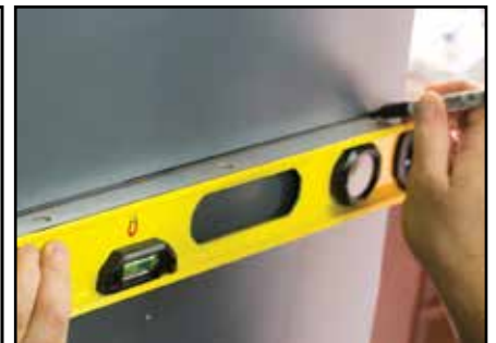
2a - Connect the marks with a level
