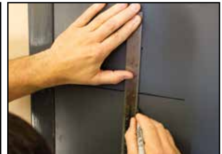
4c - Draw the vertical line from the transferred marks
