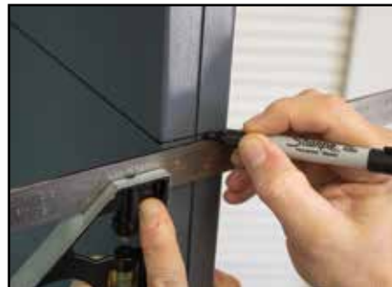
2b- Extend Horizontal line to door's edge
