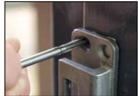
18d - Tap the slotted (top and bottom) strike holes
