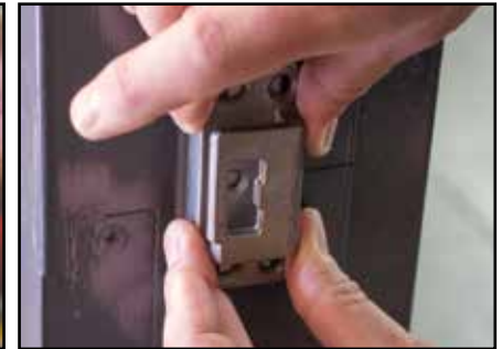
1c - Center the Strike's center hole over the 43" mark and attach.
