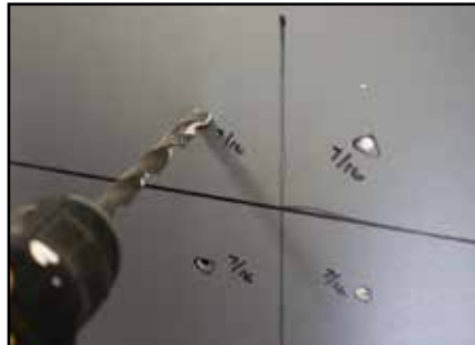
9a - Base Plate side of the door drill all (4) Exterior Trim B attaching holes
