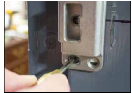
18b - Center punch the 2 slotted holes on the strike (top and bottom holes)
