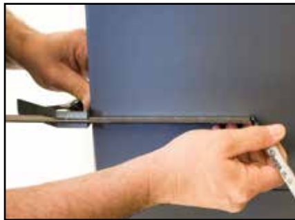
4b - Transfer vertical line to the Exterior Trim side of the door
