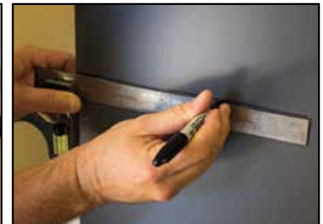
2c- Continue Horizontal line to Exterior Trim side at least 10" across the door.
